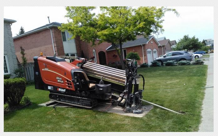
Individual drop connections that will connect homes to the network will be installed using a plow that simply makes a small slit along the ground and inserts the cable.
